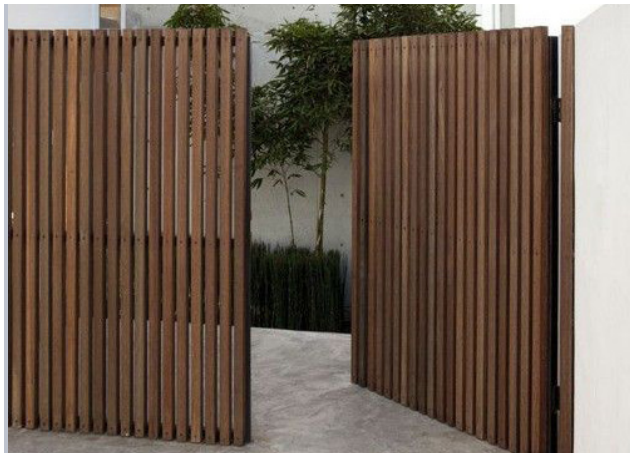
④ Timber gate - 1.6m timber semi-permeable vertical paling hinged gate. Detailed to match fence type ii
