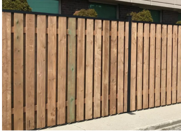
② Vertical slat open-board timber fence - 1.6m - Materials to match with closeboard fence. 150mm wide paling with 20mm spacing.
