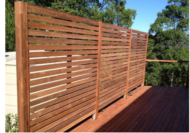
③ Horizontal slat timber screen - 1.8m - semi-permeable screen to hide service areas.
