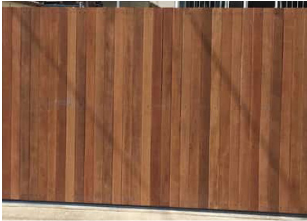
① Vertical slat close-board timber fence - 1.8m - 150mm wide paling with concrete nib at base to prevent water runoff where necessary.
